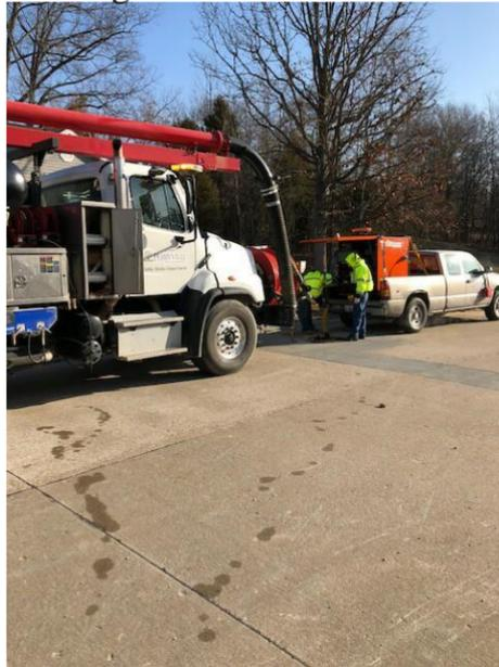
Pic(R): Cleaning and videoing Sewer mains using our Vactor and Camera equipment.
